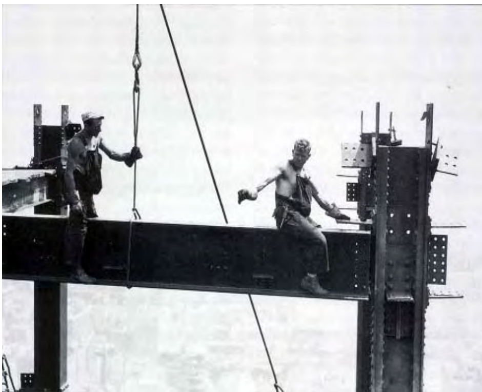
LEWIS W. HINE, STRUCTURAL STEEL (EMPIRE STATE BUILDING), ca. 1931
