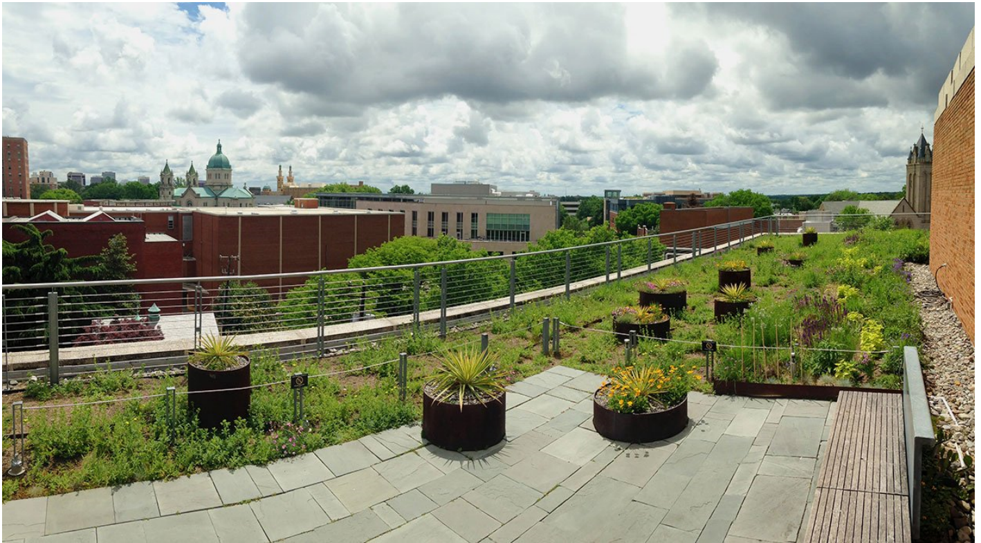
Figure 2: Virginia Commonwealth University Arts Pollak Building Rooftop Garden, Richmond, VA. 13
