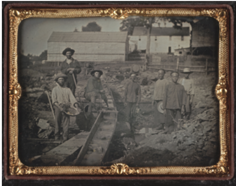
Figure 3: A Group of white and Chinese miners at a Sluice Box in Auburn Ravine, photo by Joseph Blaney Starkweather 1852.
